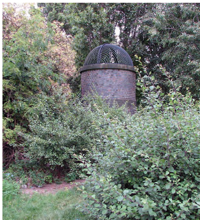
One of the ten surviving ventilation shafts. Photo Richard Griffin
